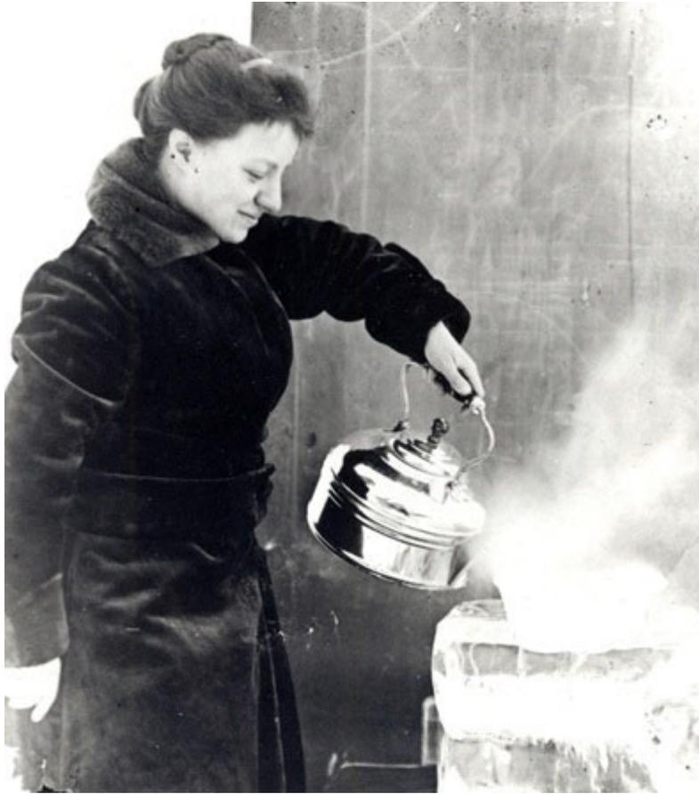
Image of Corning Glass Works laboratory physicist Evelyn Roberts, in 1917 or 1918, pouring boiling water from a teapot onto a Pyrex pie plate as it rests atop block of ice on the roof of a Corning Glass Works building to demonstrate Pyrex ware's thermal endurance. From Corning Incorporated Department of Archives and Records Management.
